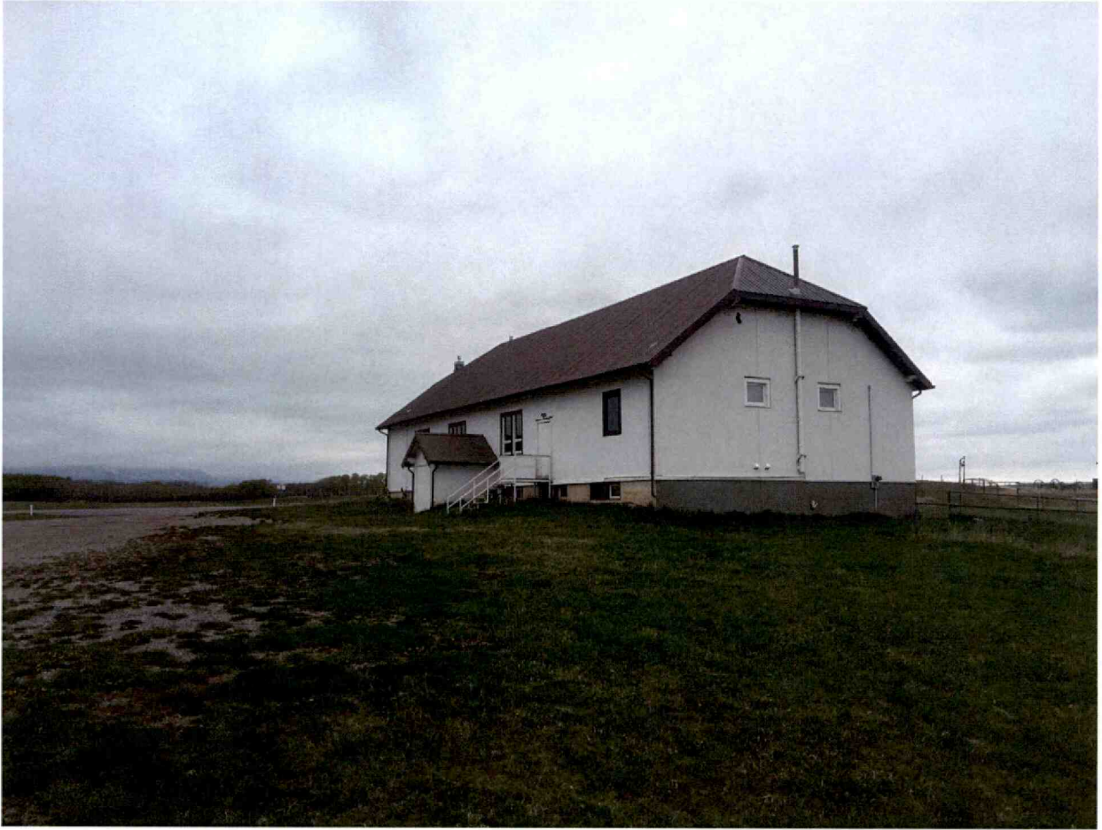
Photo 2 – Northwest from south of Hall
