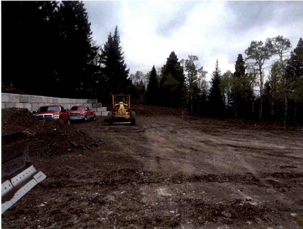
Photo 3 – Northwest at building site
