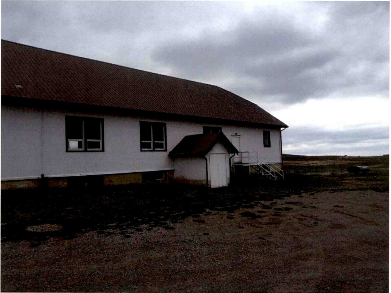
Photo 1 – Northeast from south of Hall
